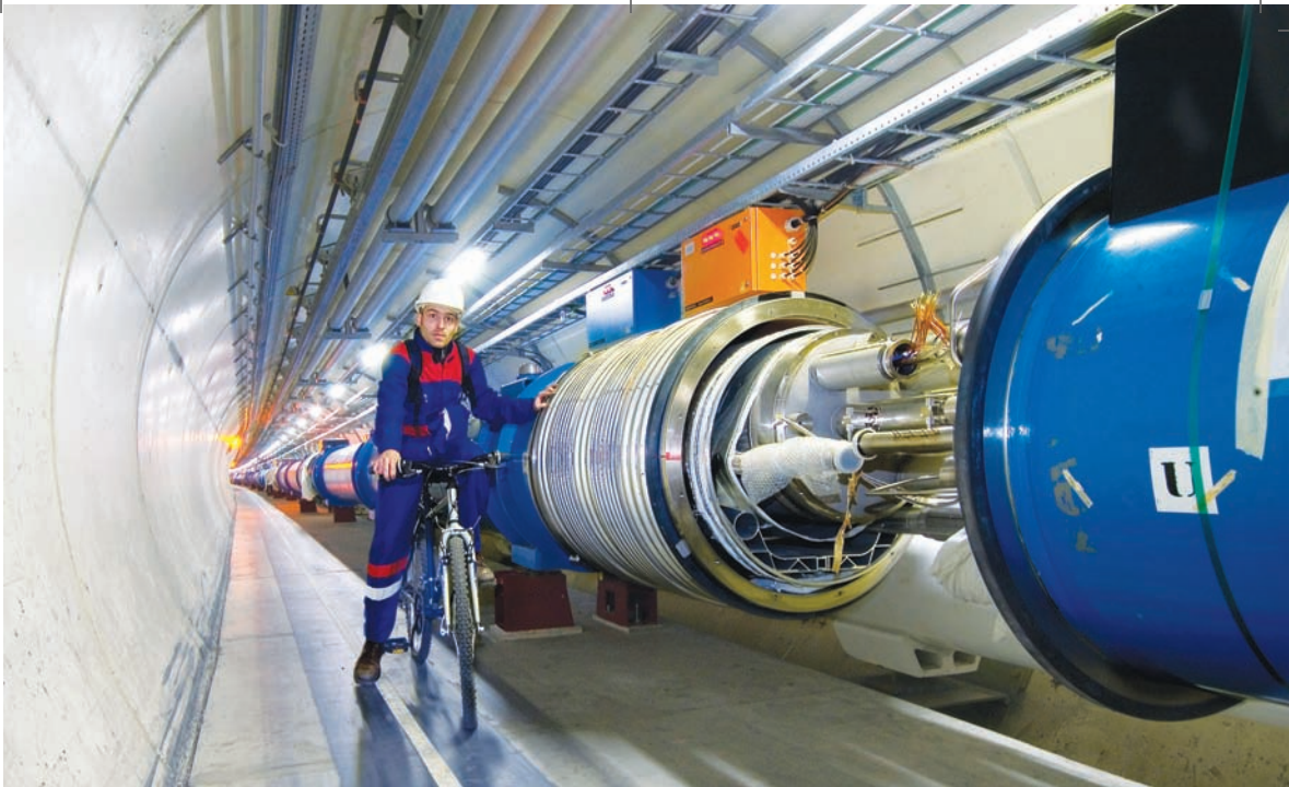
In the LHC's immense underground tunnel, 1,232 dipole magnets have been delivered to CERN and are being installed. Photo: Maximilien Brice, 24 October 2005.
